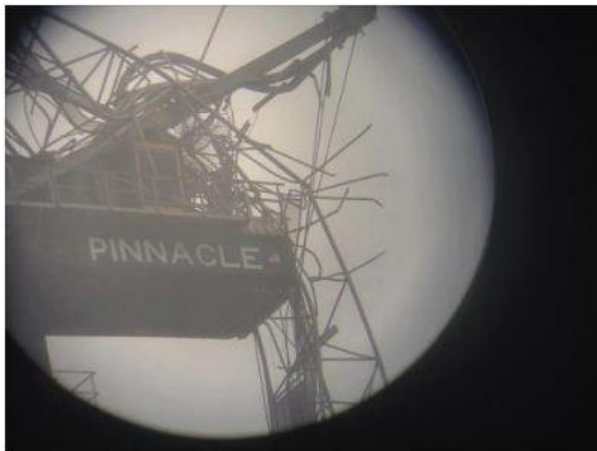
NYC Construction Crane Snaps in Hurricane Sandy, Prompting Evacuation Orders. The Story: http://abcn.ws/TqPE9E
